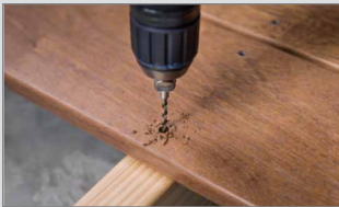
Step 1: Drill the boards and substructure with a SPAX Step drill. Use the complete length of the drill. Use the highest possible speed (around 3,000 rpm).
