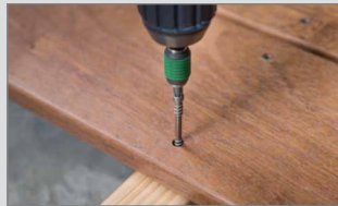
Step 2: Drive the decking screw straight in with a T-STAR plus T25 BIT. Drive it in without stopping until the head is flush.
